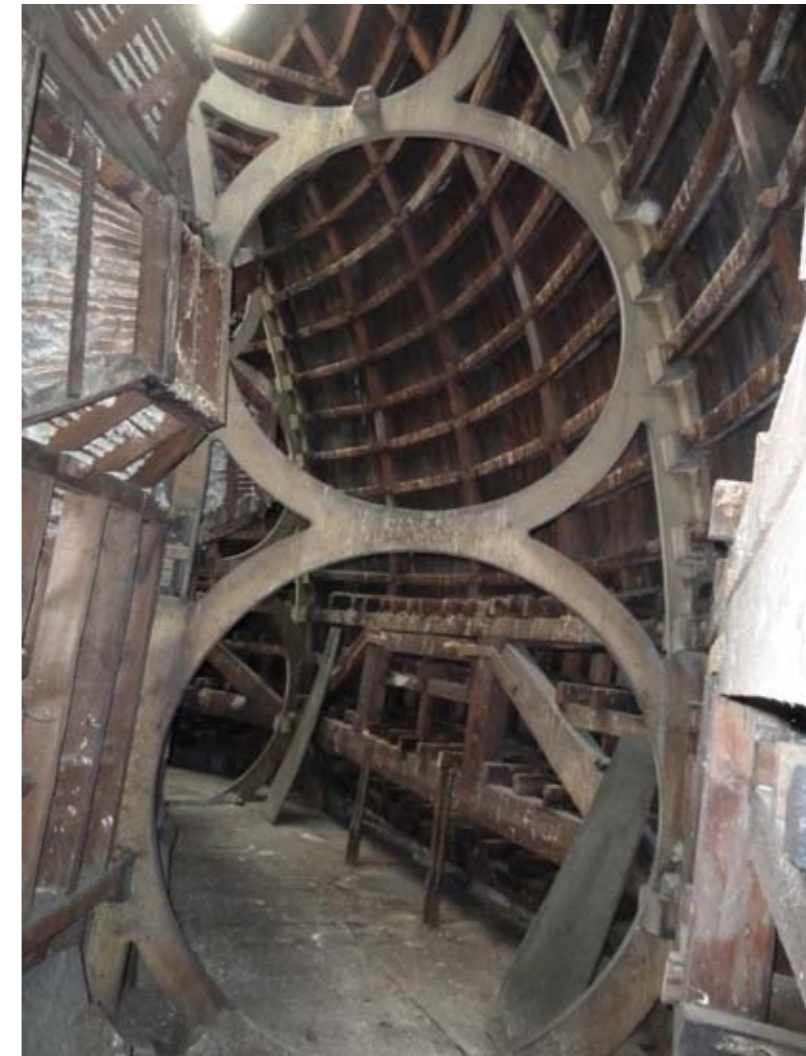
18. Chapel roof void and dome structure 2014.
